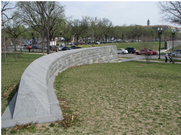
Images: completed stone-clad levee stem walls (Source Pl.’s Ex. 5)
