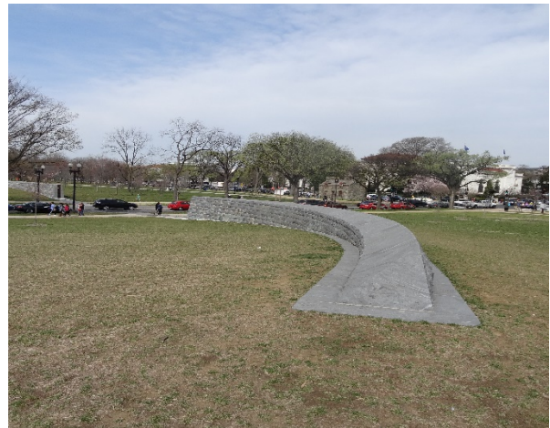
Images: completed stone-clad levee stem walls (Source Pl.’s Ex. 5)
